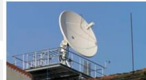
RAPIDEYE'S S-BAND ANTENNA ON TOP OF HEADQUARTERS
